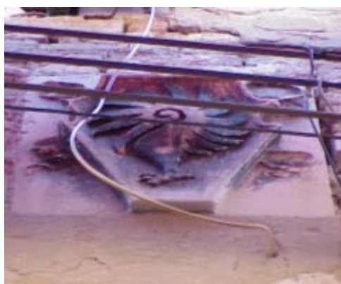
Figure 12: Wires on and around public art
