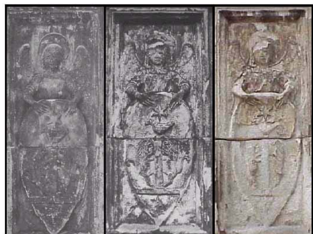
Figure 10: Public art deterioration
