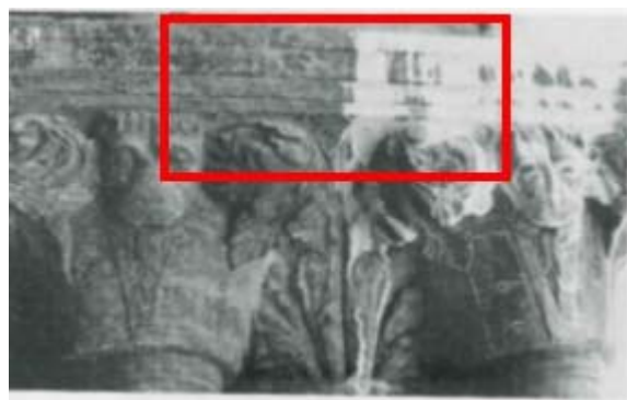
Figure 11: Blackening caused by atmospheric pollution, and whitening produced by trails of rainwater 7 .
