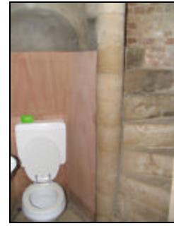
Figure 19- Restroom in Bell Tower
