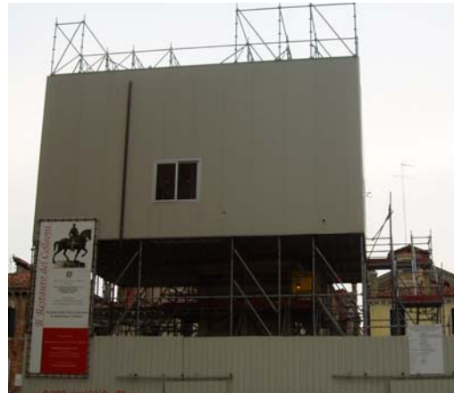
Figure 28: Example of Restoration in Progress
