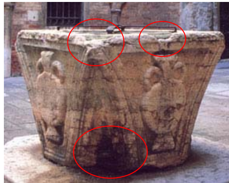
Figure 3: Example of deterioration of wells 9
