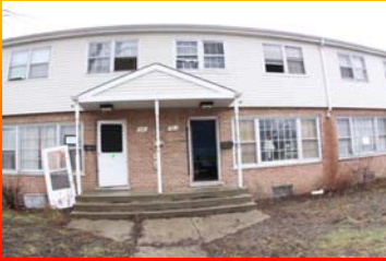
Bensenville Townhomes, scheduled for demolition
