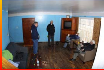
Install furnishings & instrumentation
