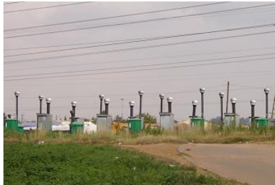
Figure 22: Enviro Loo Toilets at an Informal Settlement (Clean up America, 2009)
