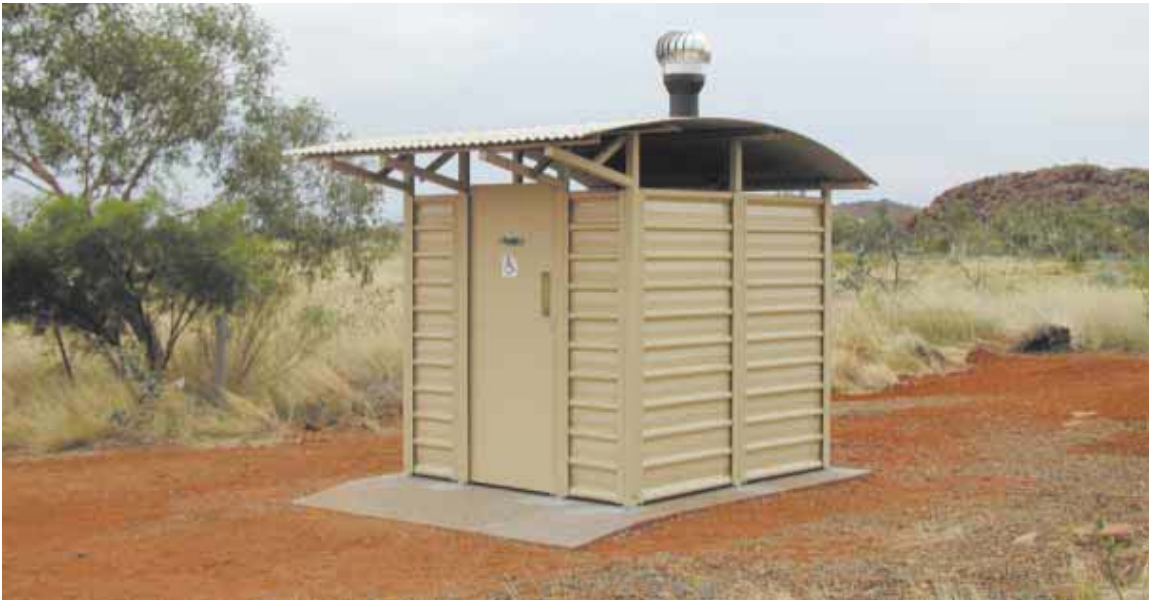
Figure 123: E-Hut construction containing Enviro Loo, specifically designed for handicapped individuals.
