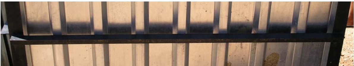
Figure 4.9: Image from Okahandja Park 1, showing 10.5 waves per sheet.
