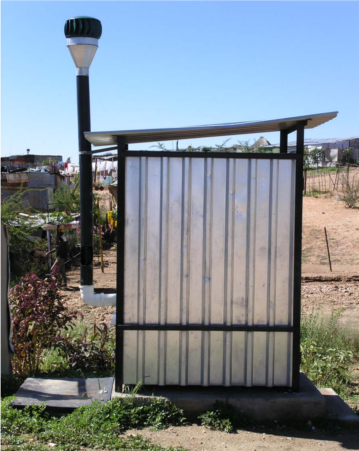
Figure 4.1: Cool Maintenance individual dry toilet facility constructed in Okahandja Park 1.
