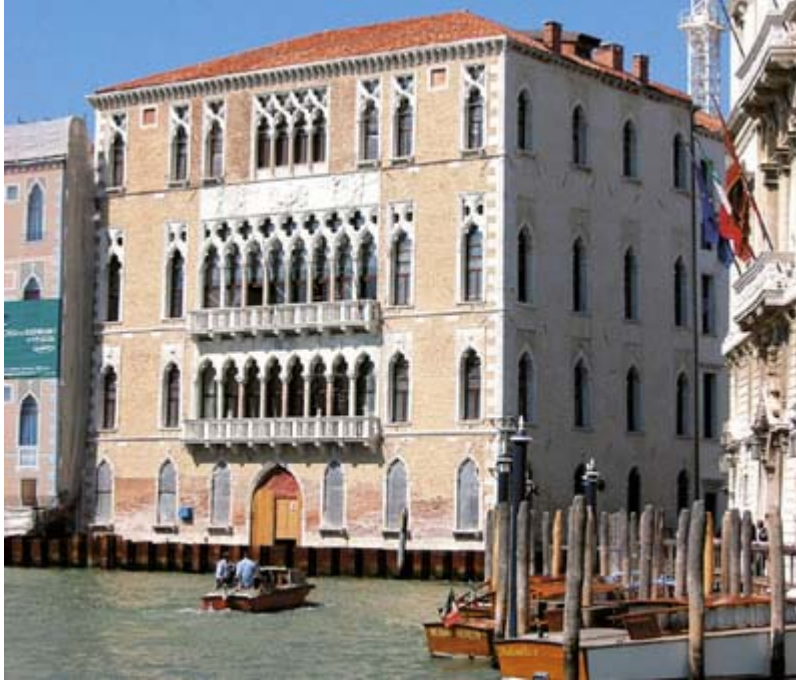
Figure 2.4: Ca Foscari after repairs
