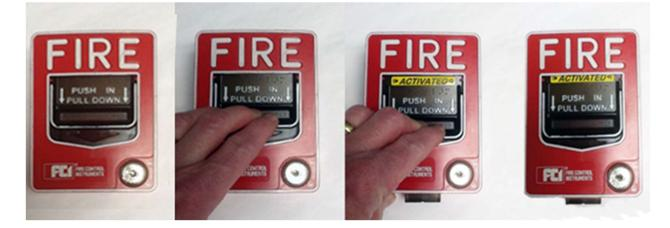
This newer style fire alarm pull station requires that you push in and then pull down. Please note - the "Activated" sign will appear when the device has been triggered.
