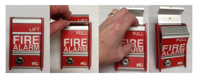
To activate this type of fire alarm pull station, lift up the flap, grasp the top of the device and pull towards you. You will hear a click, and the device will lock into position.
