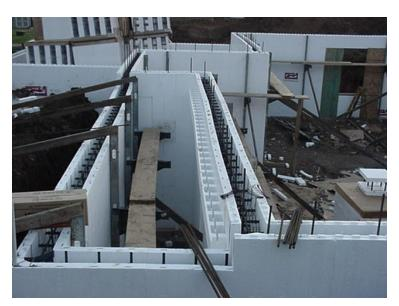
Utilizing ICF's for foundation building can improve efficiencies, save time on installation, and act as a barrier for losses through conduction. When pouring the floor, a 6 mil vapor barrier should be placed directly into the concrete. This will prevent water
