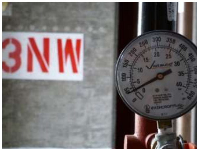
Figure 3.21. Floor 3 control assembly
