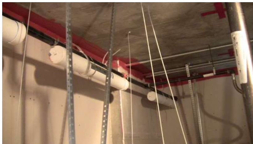
Figure 3.11. Sand weight on Floor 1 sprinkler pipe in the EL area
