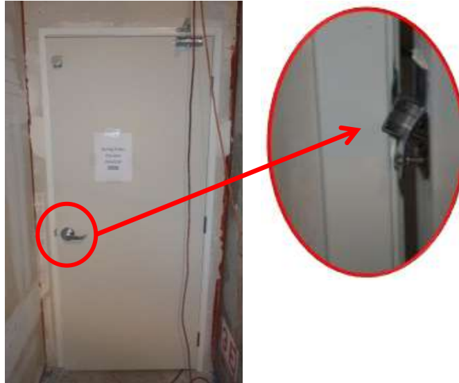
Figure 5.7. Corridor door jam
