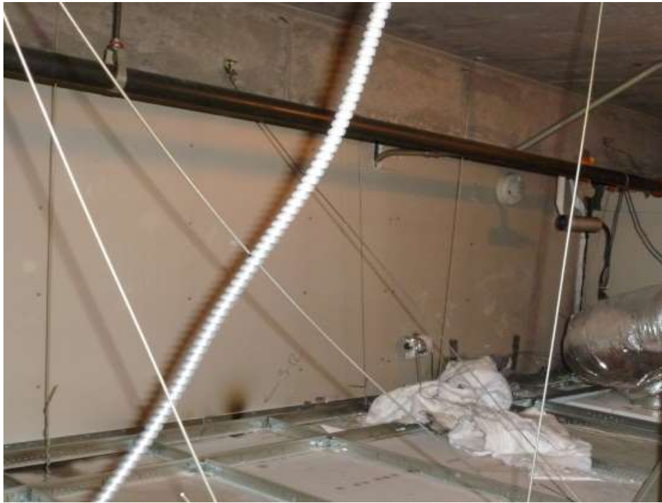
Figure 8.30. North wall of LBR above the ceiling after LBR-2 fire test
