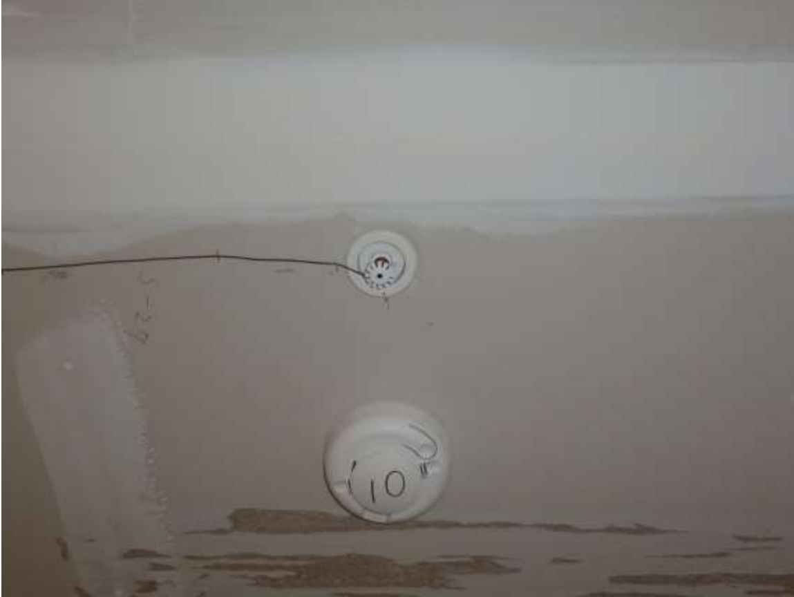
Figure 7.15. Smoke Detector 10 installed on the SBR ceiling
