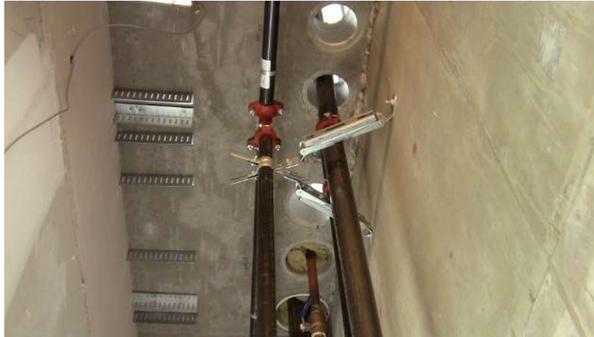
Figure 3.10. Seismic bracing on Floor 1 main feed
