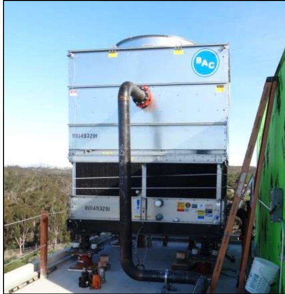
Figure 2.16. Cooling tower in the roof
