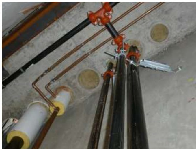
Figure 3.23. Seismic bracing on Floor 3 main feed
