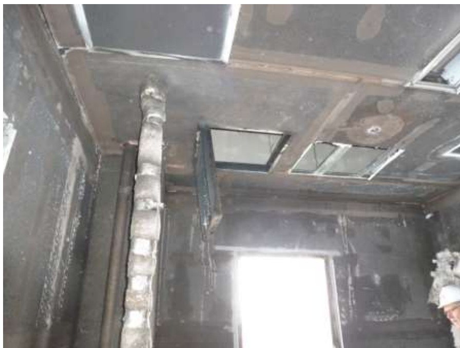
Figure 7.42. Portion of the ceiling cut off adjacent to the access panel
