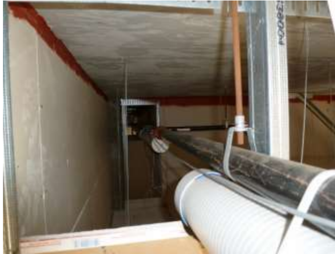
Figure 3.33. Sand weight on Floor 4 sprinkler pipe in the EL area
