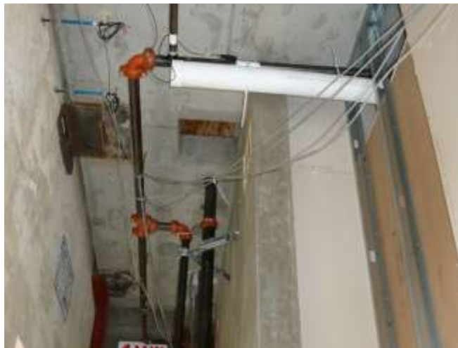
Figure 3.30. Seismic bracing on Floor 4 main feed
