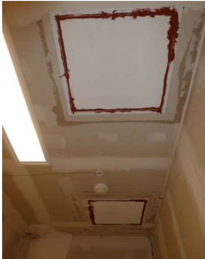
Figure 7.30. SBR ceiling vent blocked with ceramic fiber board
