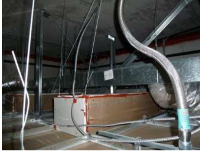
Figure 3.26. Flexible drop on Floor 3 3C LBR sprinkler head
