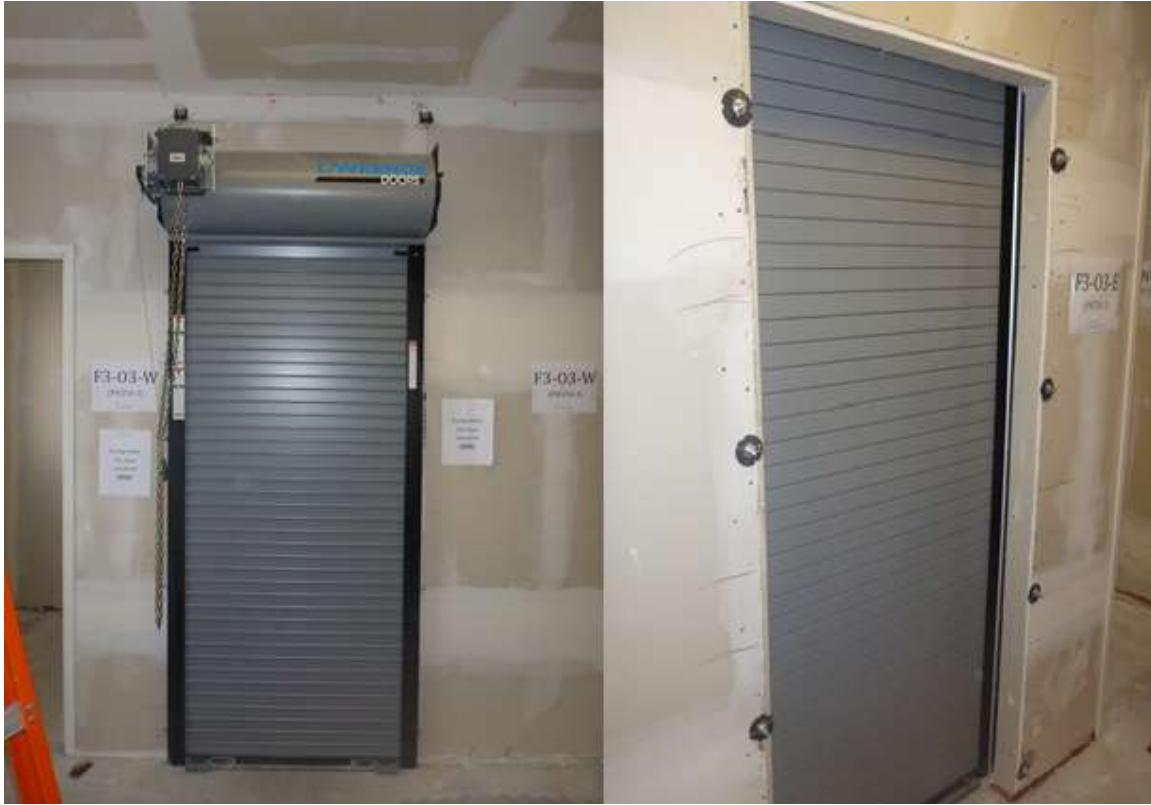
Figure 3.61. Front and back of fire door when rolled down
