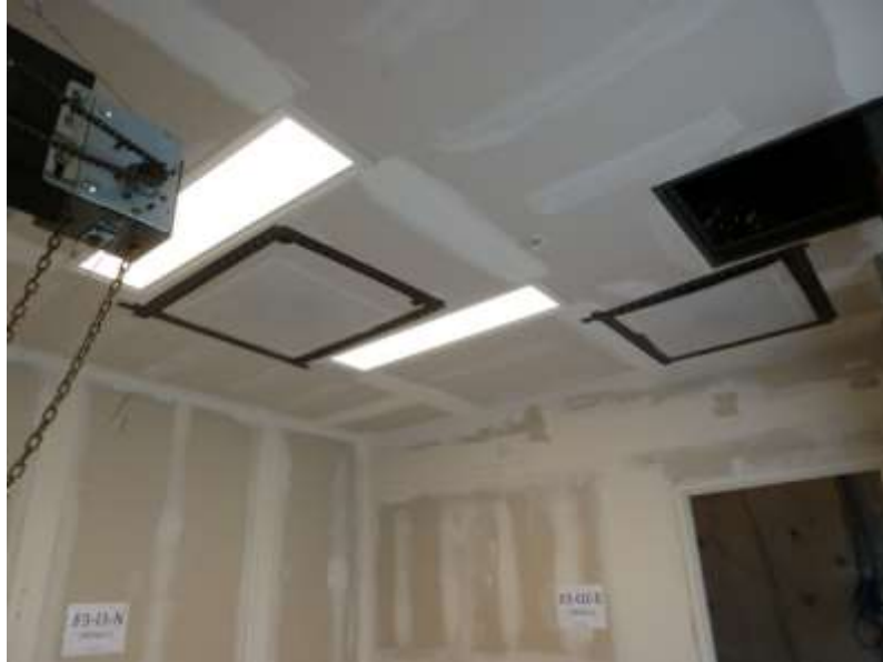
Figure 2.8. Floor 3 finished ceiling system with vents and access panel
