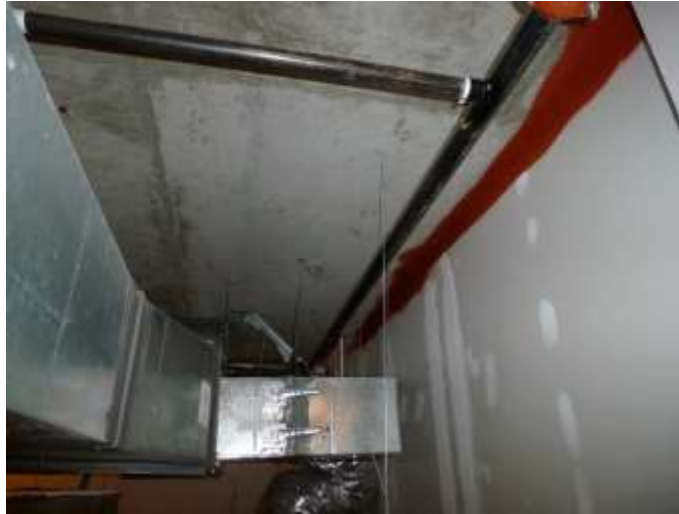
Figure 3.24. Seismic bracing on Floor 3 EL area sprinkler pipe
