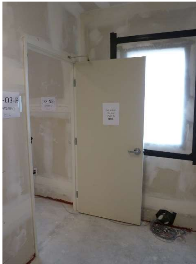
Figure 3.67. Door 1, particleboard core door
