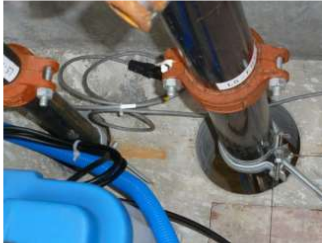
Figure 3.39. Clamps on bottom of Floor 5 riser and drain pipe
