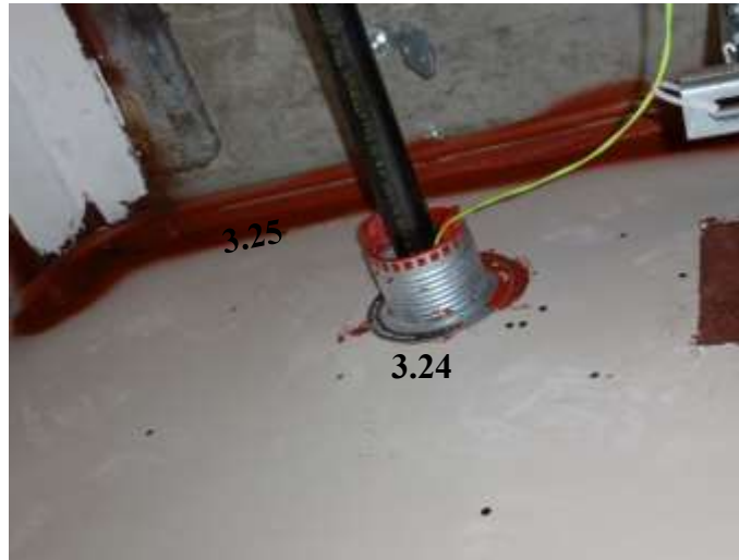
Figure 3.52. Floor 3 corridor and LBR pipe penetration
