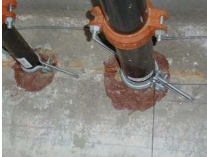
Figure 3.22. Clamps on bottom of Floor 3 drain pipe and riser
