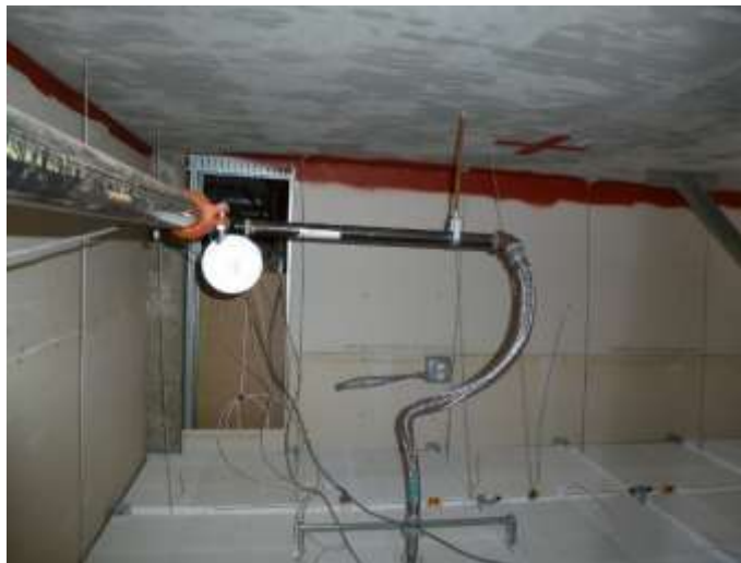
Figure 3.34. Flexible drop on Floor 4 4A sprinkler head
