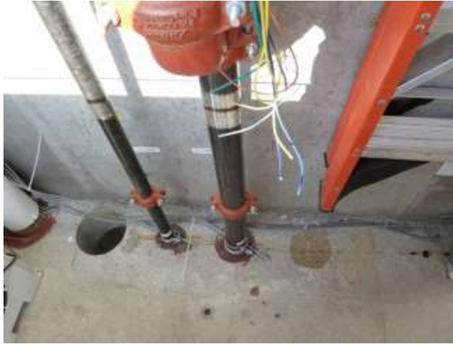
Figure 3.29. Clamps on bottom of Floor 4 drain pipe and riser
