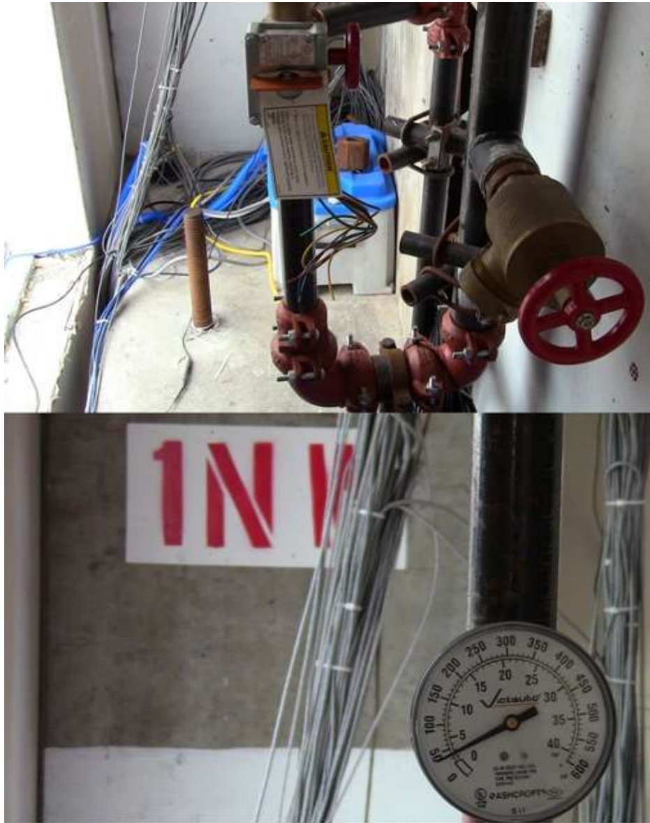
Figure 3.8. Floor 1 control assembly
