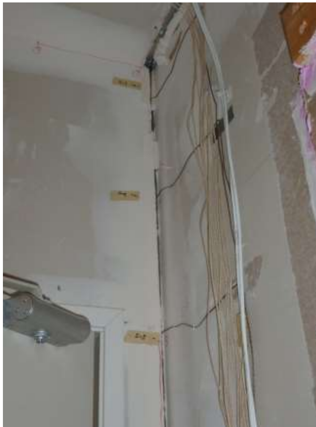
Figure 5.3. Gap formed on the partition wall between LBR and SBR
