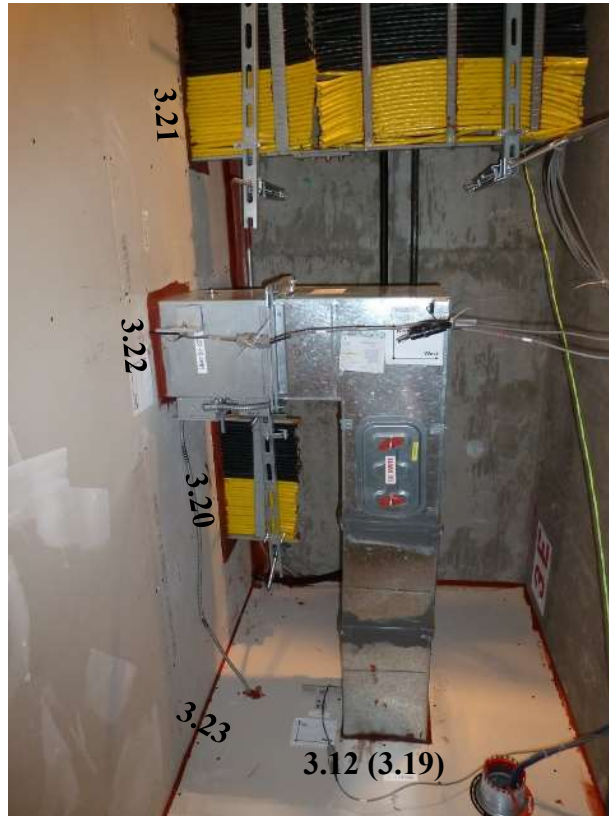
Figure 3.51. Floor 3 corridor firestop
