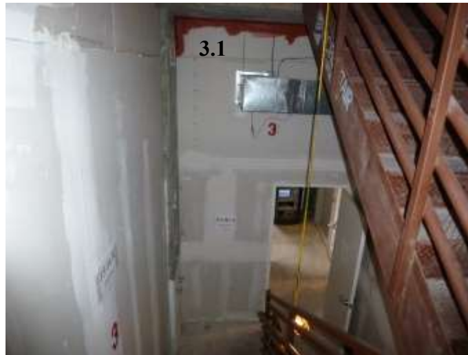
Figure 3.43. Floor 3 landing wall-slab gap firestop
