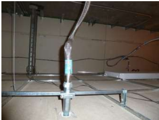
Figure 3.13. Flexible drop on Floor 1 EL sprinkler head
