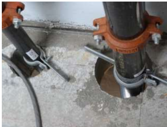
Figure 3.17. Clamps on bottom of Floor 2 drain pipe and riser
