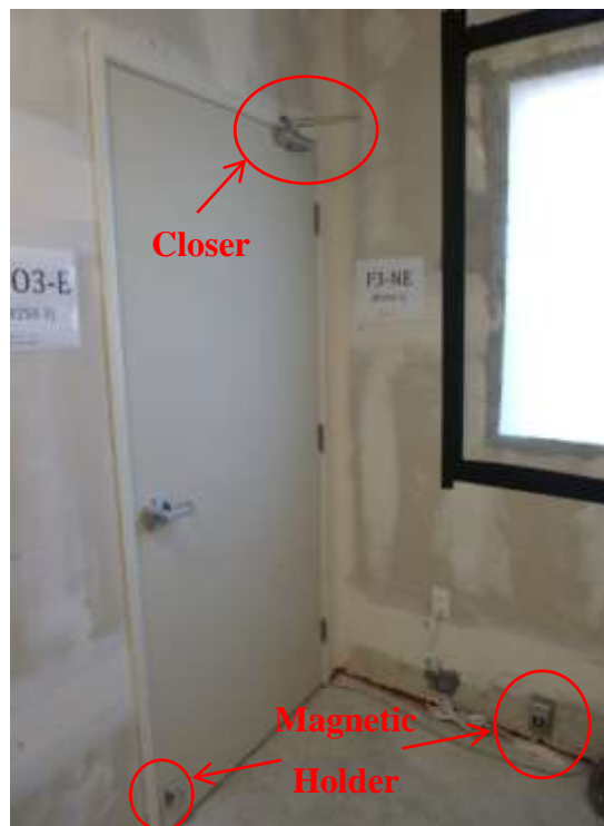
Figure 3.68. Door closer and magnetic door holder
