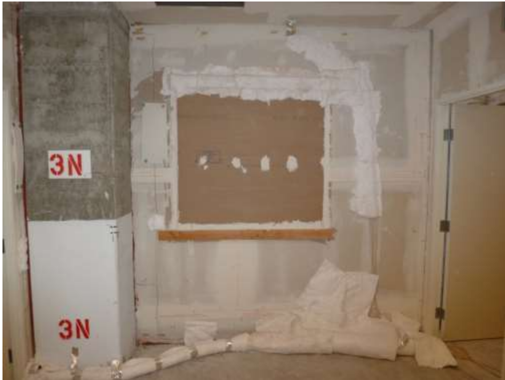
Figure 7.25. LBR window blocked with wood panel
