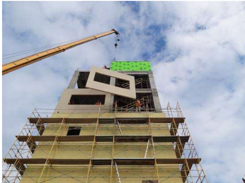
Figure 2.4. Installation of concrete panel on the 4 th floor
