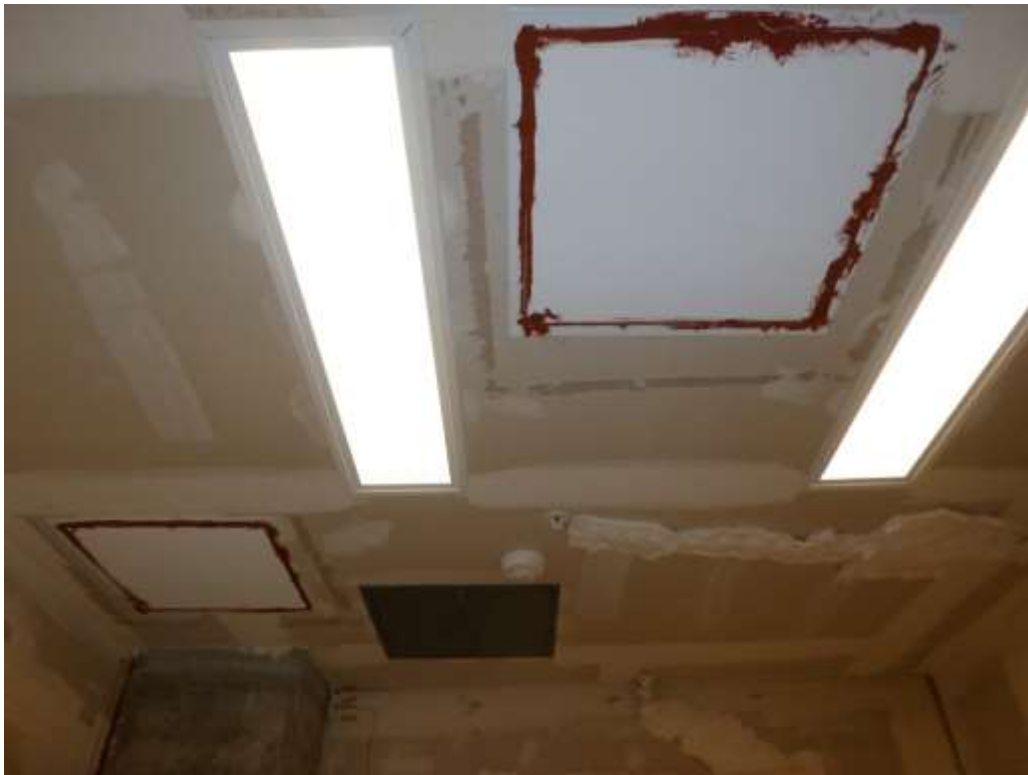
Figure 7.26. LBR ceiling vents blocked with ceramic fiber board
