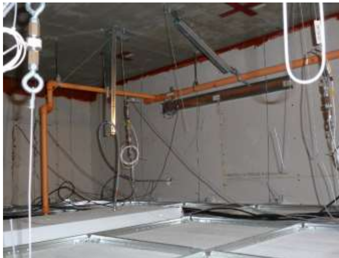
Figure 3.19. Seismic bracing on Floor 2 EL area sprinkler pipe
