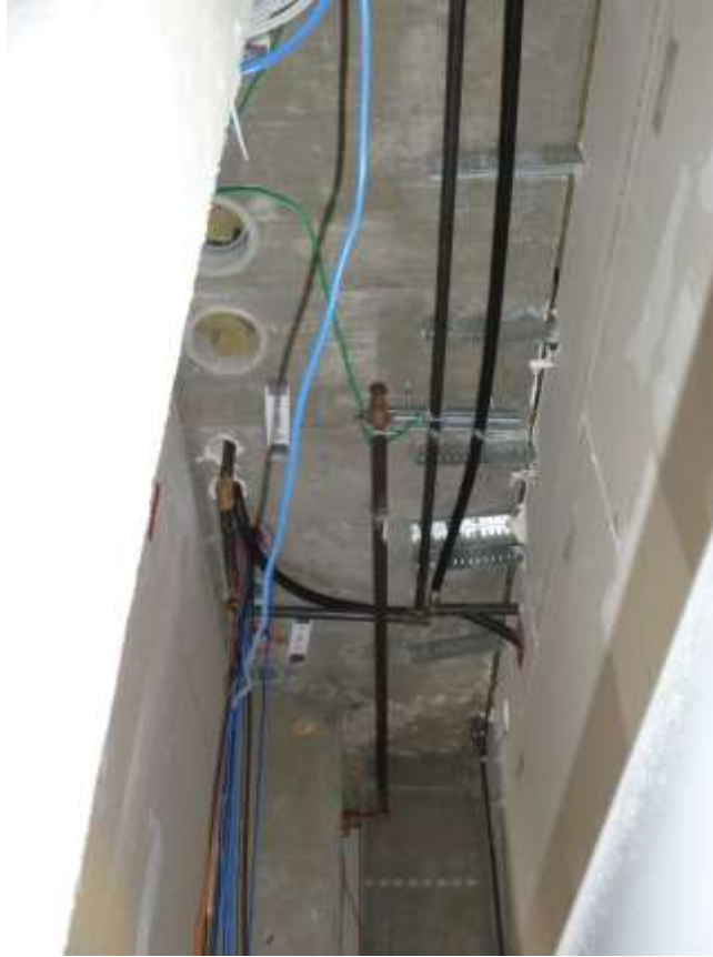
Figure 6.3. Floor 1 rigid gas pipe disconnection
