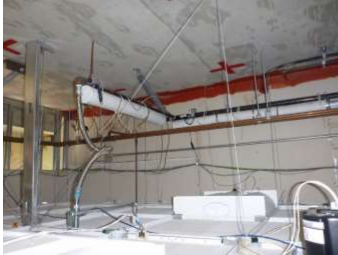
Figure 3.35. Flexible drop on Floor 4 4C sprinkler head
