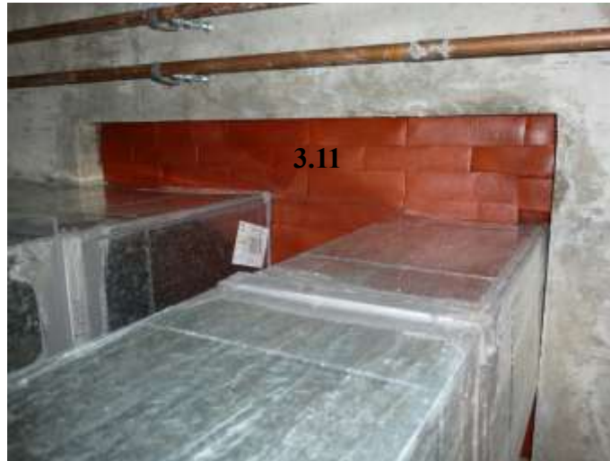
Figure 3.48. Floor 3 vertical firestop for vent penetration above ceiling of EL (EL view)
