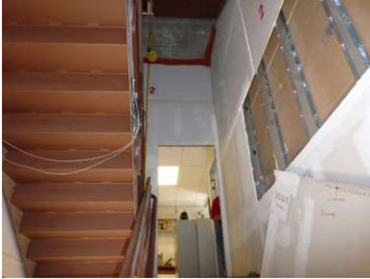
Figure 6.6. Wallboard detachment following FB-6 around intermediate landing of Floor 1 and 2
