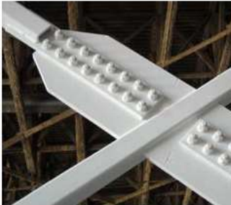
Cross bracing protected with intumescent coating
