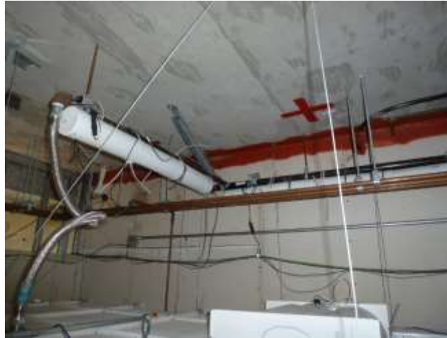
Figure 3.31. Seismic bracing and sand weight on Floor 4 sprinkler pipe in the eastern room area
