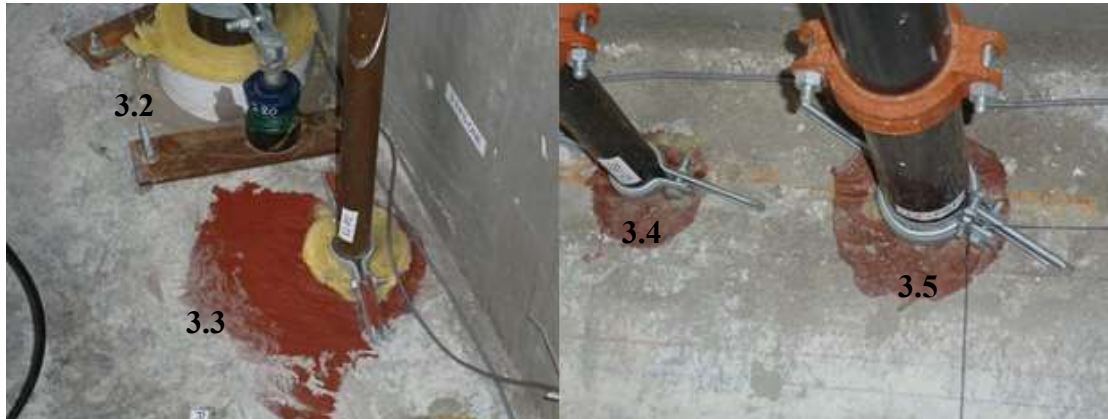
Figure 3.44. Floor 3 west side of shaft penetration firestops
