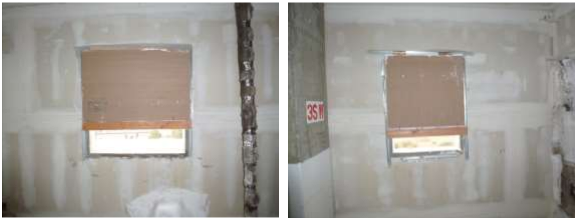
Figure 7.39. EL windows blocked with wood panels
