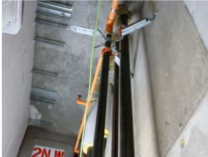
Figure 3.18. Seismic bracing on Floor 2 main feed
