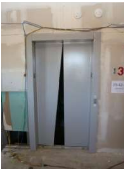
Figure 5.8. Damage to the elevator door in Floor 3
