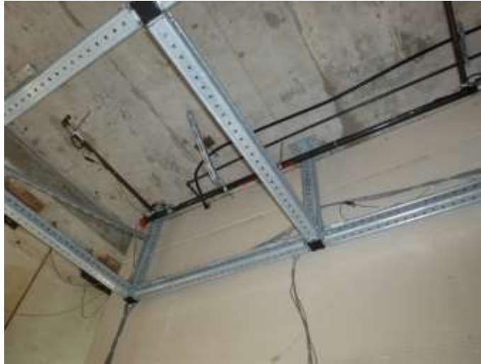
Figure 3.41. Seismic bracing on Floor 5 branchline pipe running across the room area
