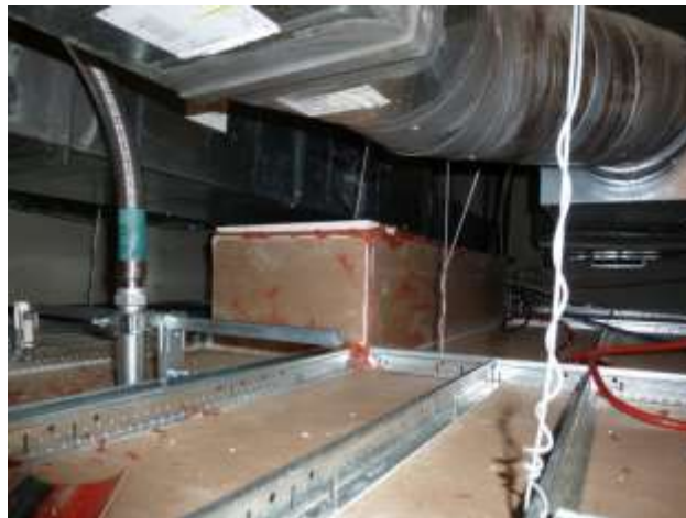
Figure 3.25. Flexible drop on Floor 3 EL 3A sprinkler head
