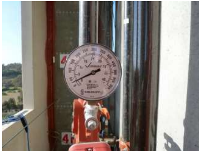
Figure 3.28. Floor 4 control assembly
