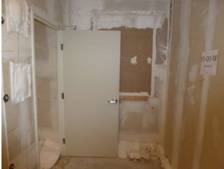
Figure 7.29. SBR window blocked with wood panel
