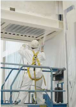
Typical Hilti Fire Protection Steel Spray application
