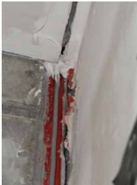
Figure 5.5. Gaps in the joint area of Floor 3
