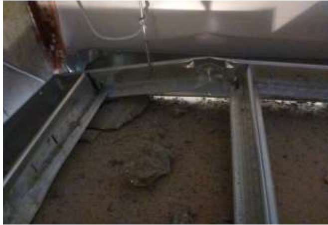
Figure 5.4. Gap formed in the north wall balloon framing in the joint area above the LBR ceiling
